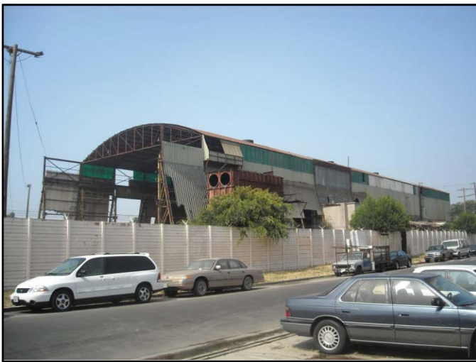
View of abandoned steel mill on HACLA-owned property.
